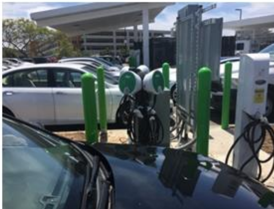
Charging Island Side View Two chargers per pedestal – 4 total for 3FCA and 1Honda PHEV
